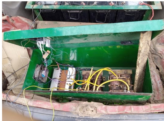
Plate 3: Installation of inverter
