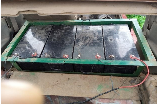
Plate 2: Installation and connection of batteries
