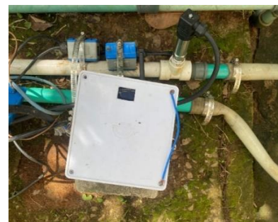
Figure 4: Device installation along pipeline
