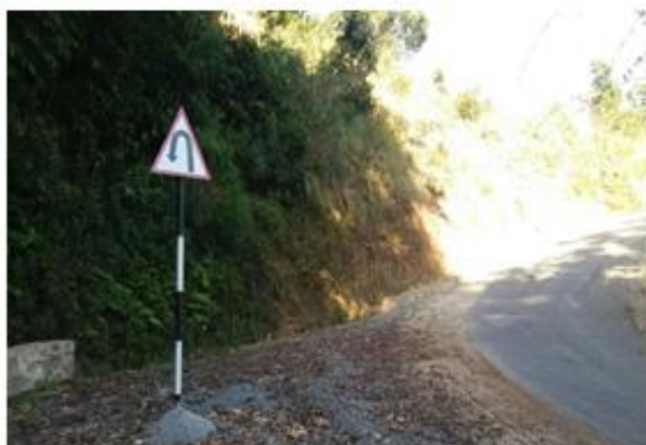
Fig-3: Installation of Traffic Sign and Delineator post
