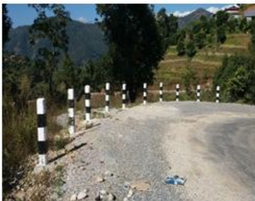
Fig-3: Installation of Traffic Sign and Delineator post
