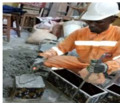
b) Placement of concrete mix in mould
